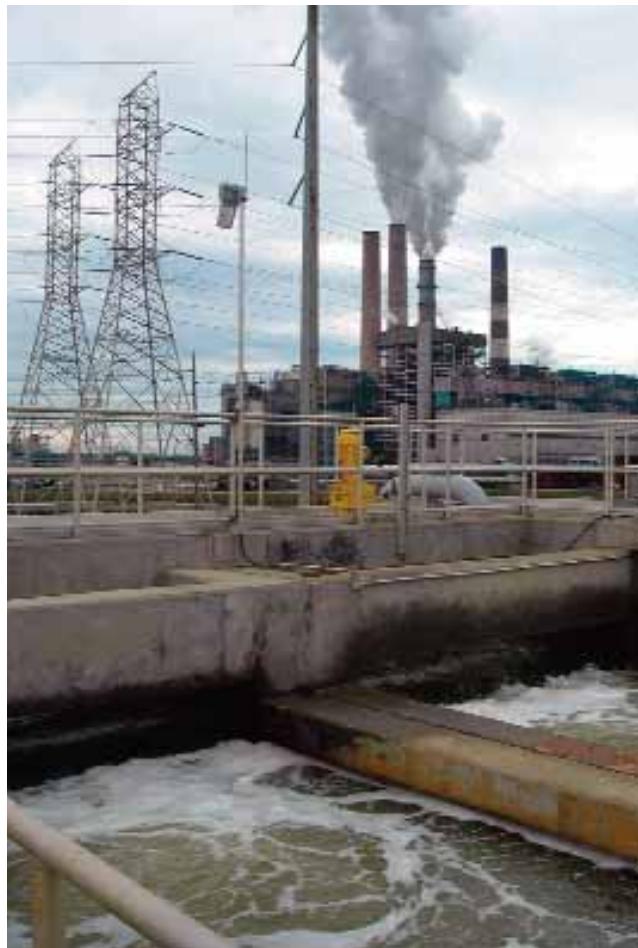
Desalination plant in Tampa, Fla., and the electrical generating plant that powers it.
