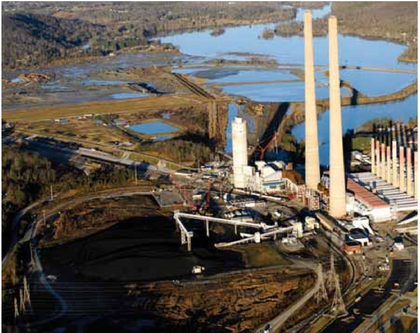
The destructive wave of coal ash that breached its containment (upper left) at the TVA's Kingston Fossil Plant was photographed by Dot Griffith, with aviation assistance from SouthWings ( www.southwings.org ). For more about Griffith's experience, see: http://freakonomics.blogs.nytimes.com/2009/01/08/the-tennessee-coal-ash-spill-in-pictures ). Photo © Dot Griffith Photography.
