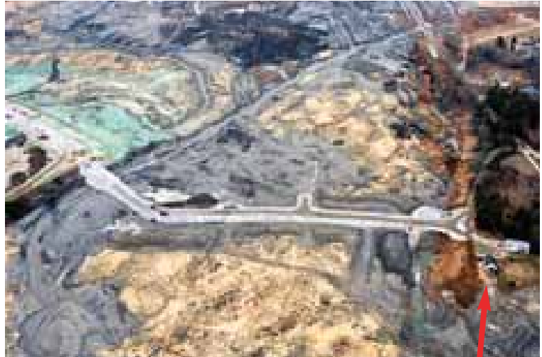
Two months after the spill, a dike constructed to prevent further contamination of the Emory River is nearly complete. (The house on the cover appears severely damaged, but still standing in the lower right-hand corner.) Photo courtesy TVA.
