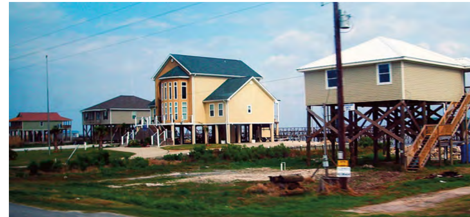
A row of elevated houses in New Orleans.
