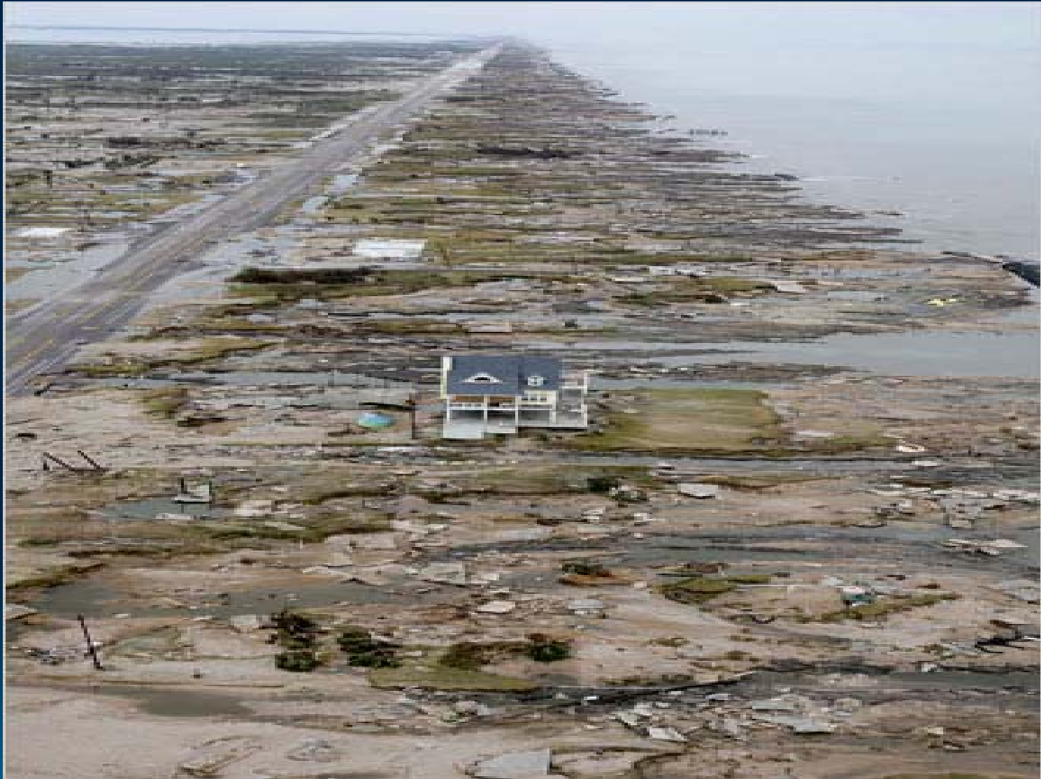
Bolivar Peninsula, Texas Hurricane Ike, Category 2, September 2008
